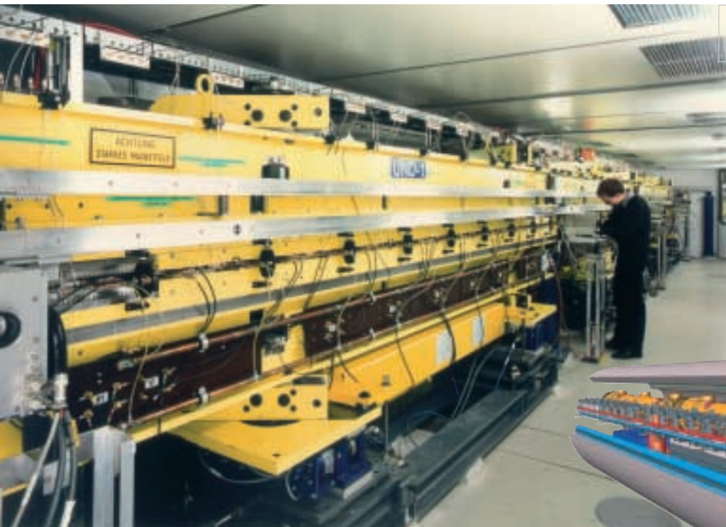
The free-electron laser under construction.
